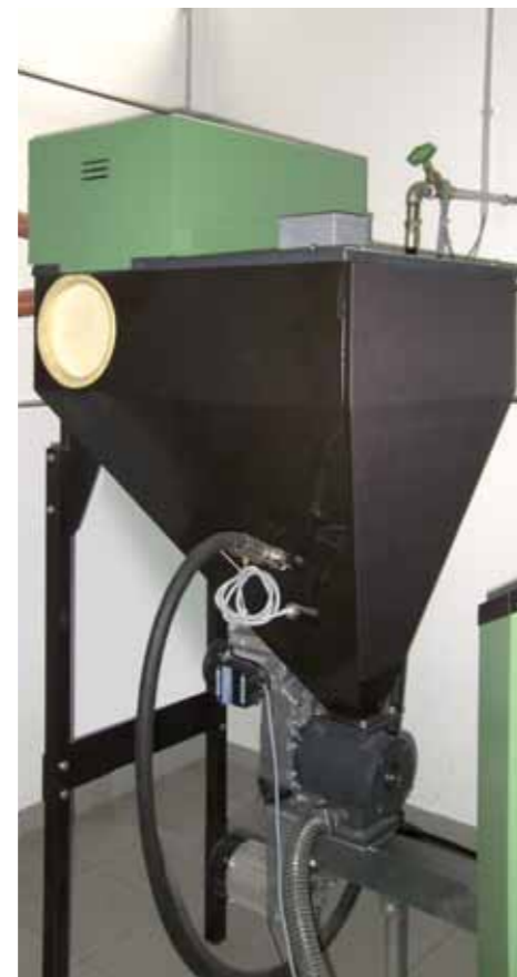
The intermediate container of the HDG pellet suction system can hold up to 100 kg of pellets. This quantity is sufficient to operate the HDG Compact 50 for over 8 hours without needing to be refilled.
