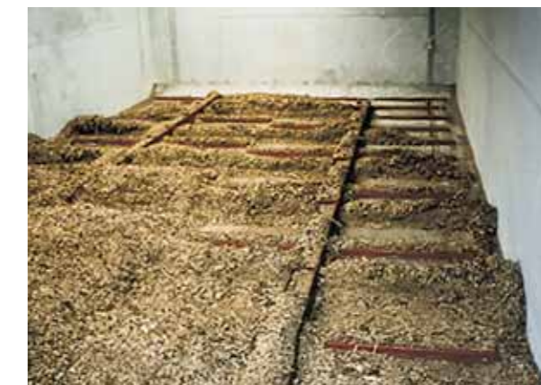
The HDG sliding tray delivery system is often used for larger heating systems. It has the greatest loading volume.
